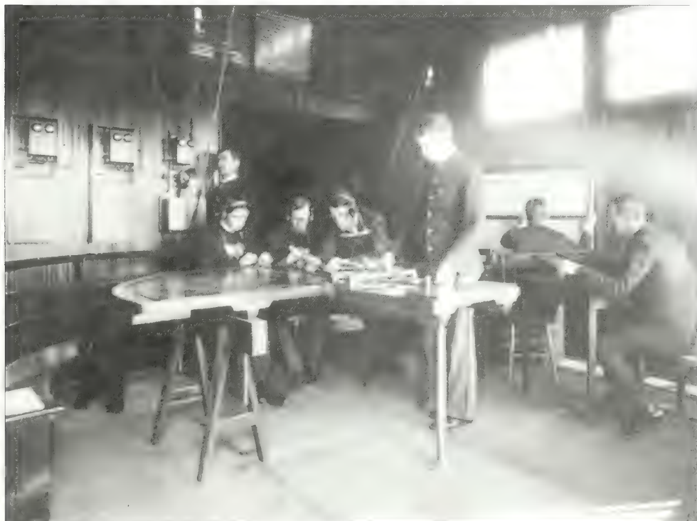
Figure 2.25. Interior of Battery Potter plotting room, circa 1907. Part of the Taft Board's recommendations to incorporate the latest technology resulted in improvements to fire control—the process of acquiring and firing on enemy ships. The communications between observation, calculating, and firing were increasingly handled by telephone, seen mounted on the wall in this image (GATE 7819).
